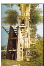
Dipping Platform - Constructed of sustainably produced hardwood with removable barrier to allow pond dipping
